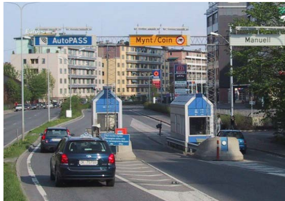
Before 2008: manned and automatic toll plaza
